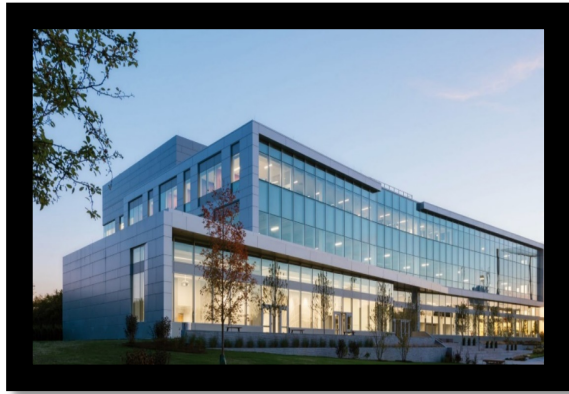
Building 5 147 South Bedford Street
